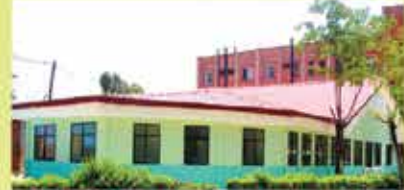
Prefab Hospital Made Up Of Cement based Prefab Panel with MS Steel Structure
