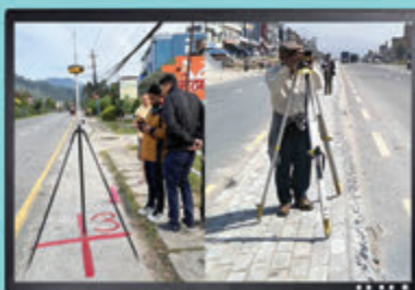
GNSS Survey & Leveling
